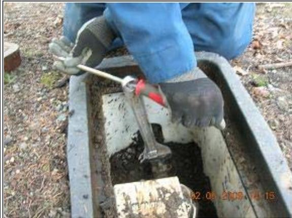
To turn the meter back on, reverse the process. Turn the meter stop slowly to allow the water to gradually return into the water line. When the arrow on the top of the meter stop points towards your house, the meter is on and you will once again have water supply in your home
