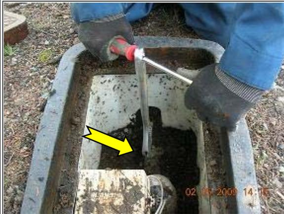
Stand the crescent wrench on the meter stop and insert your screwdriver through the hole in the end of your wrench to form a "tee". Then turn the wrench one clockwise 180 degree turn to the "off" position. When the "ears" on the meter stop line up, and the arrow on top of the meter stop points toward the street, the meter is off.
